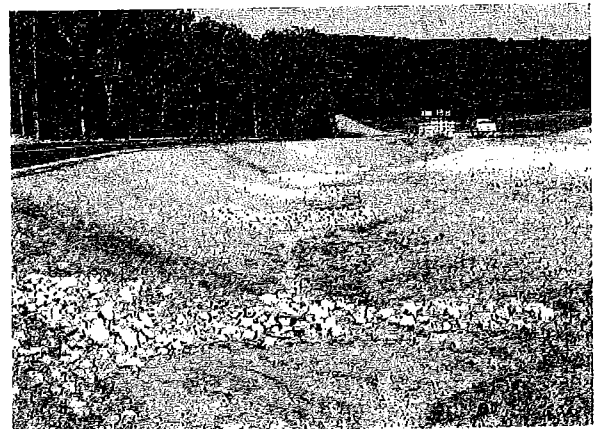
Figure 1. Silt Fences are placed at the perimeter of the job site to capture and prevent sediment from leaving the site.
